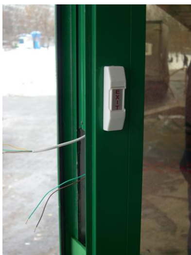
Mounting the "Exit button" onto the door (door-case) surface
