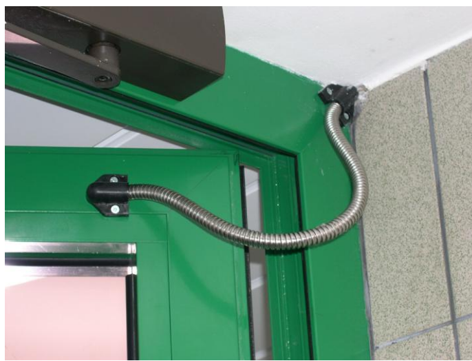
Mounting the flexible metal hose
